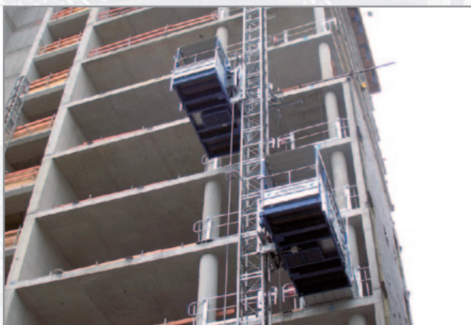
Superlift LX 2024 – A34 in twin-platform operation
