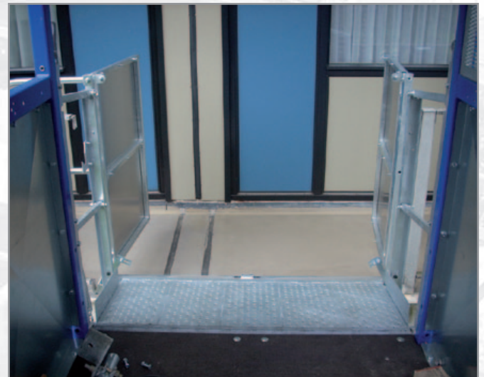
Landing with opened platform ramp
