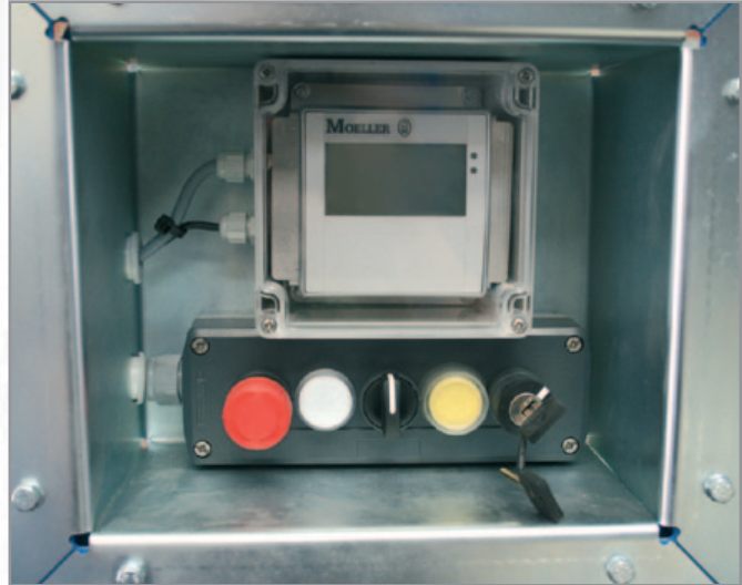
Control via convenient rotary switch
